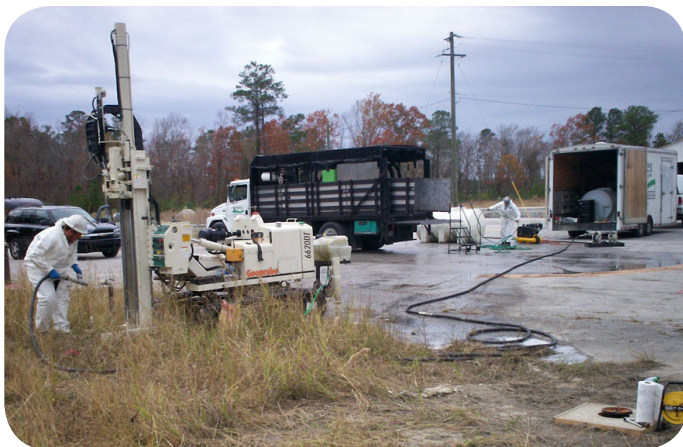
Injection of reducing agent into a hole drilled underground.
